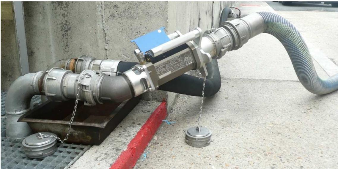
*Improper rotation/longitudinal axis*
